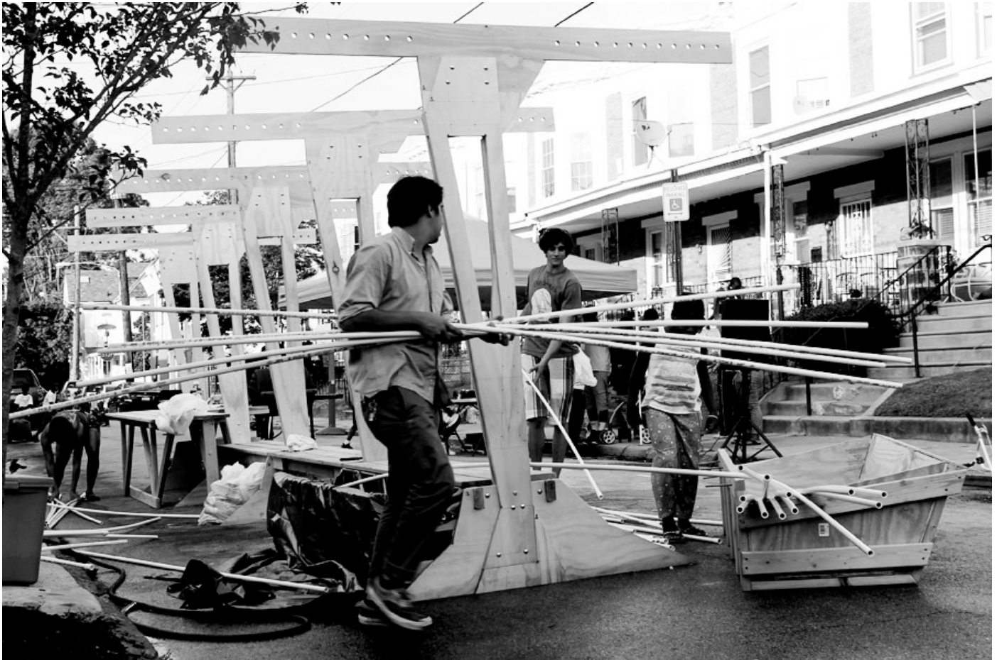
Figure 3: Construction of bays, canopy, and troughs
